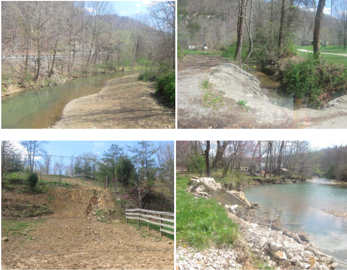
Figure 3.16. Photos from the Christy Creek Watershed, CC-2.00.
