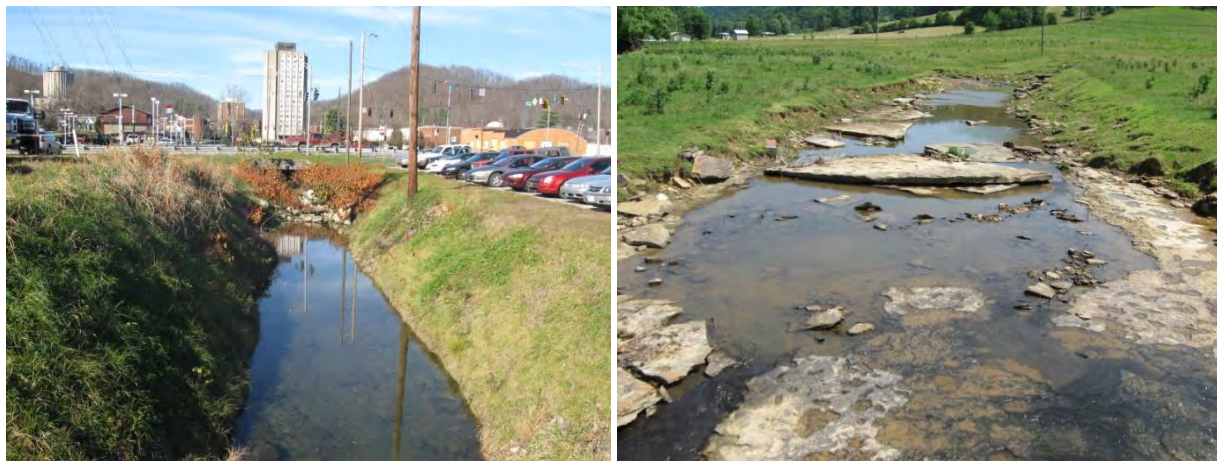
Figure 3.47. Photos of the two worst sites, EB-0.04 (left) and IF-0.05 (right).
