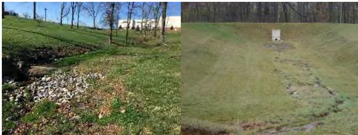
Existing storm water management features on Gateway Campus to be redesigned and improved.
