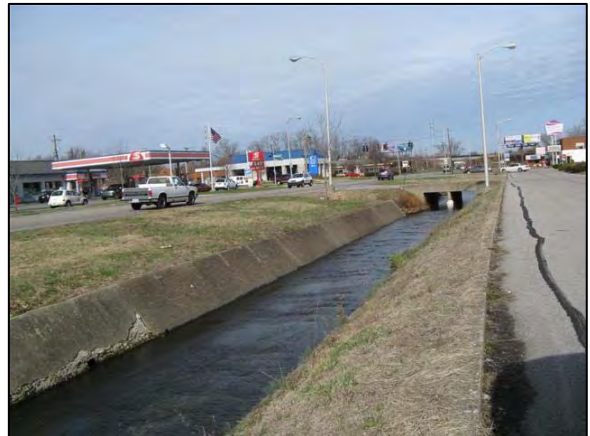
Wolf Run, Concrete Channel Beside Southland Drive
