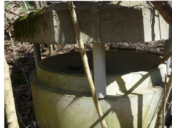
“Overflow” Structure (Before)
