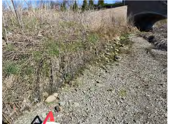
CR4- Bank Stabilization (b)
