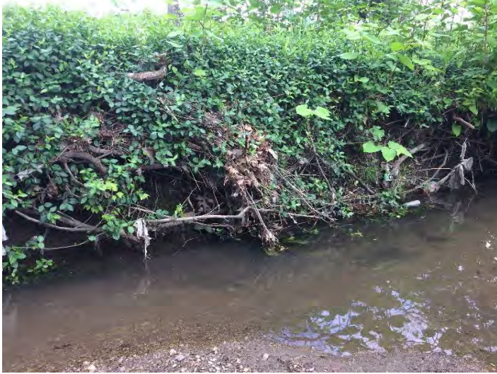
G2- Undercut Bank Root Mat
