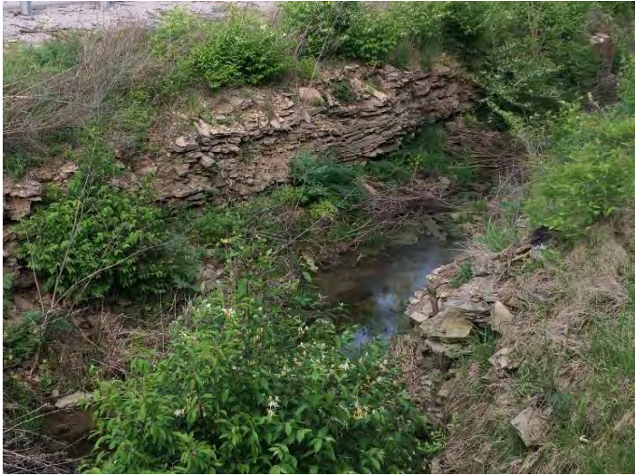
AI- Bank Undercuts (Rb)
