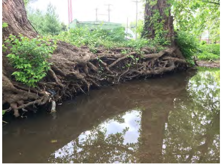
G2- Root Mat Undercut Bank
