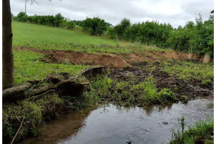
ES-11, Erosion due to cattle access
