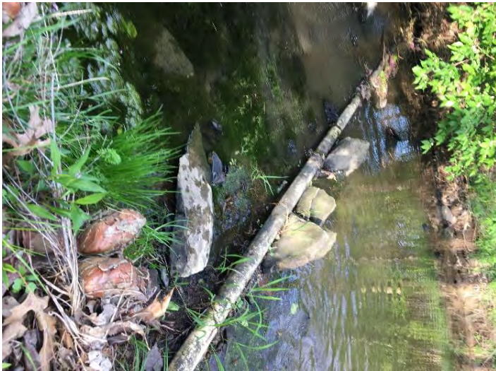
D2-Pipe Crossing Creek
