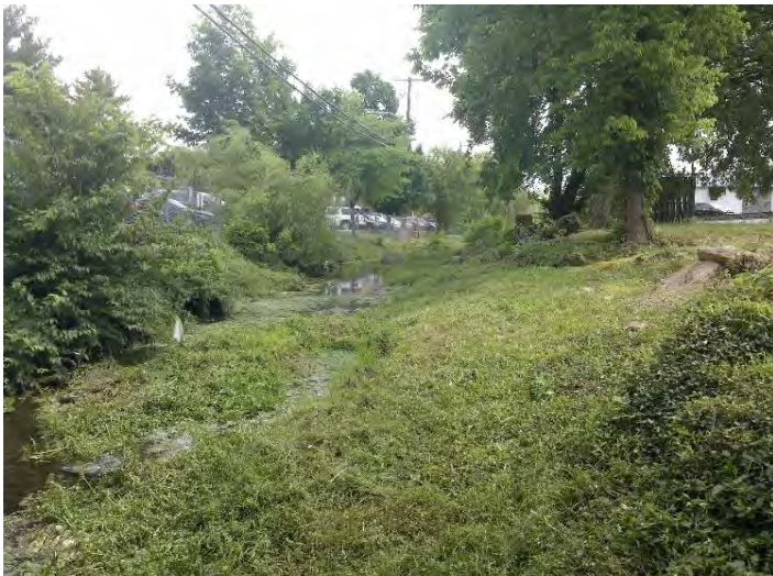
CR7- Downstream View from Upstream End of CR-7
