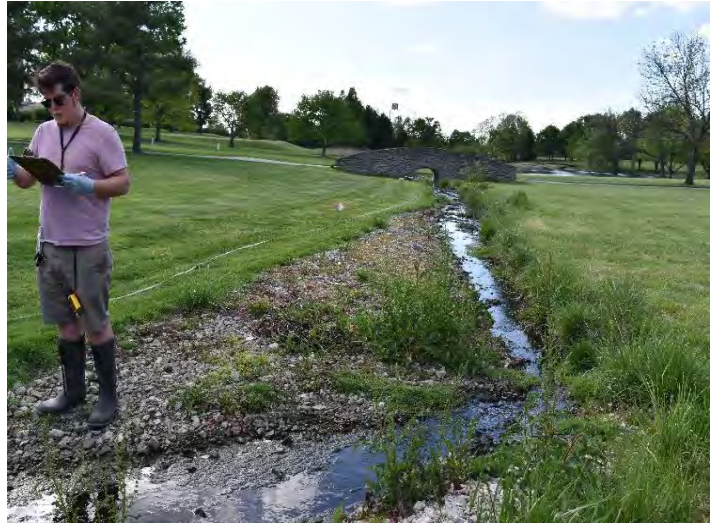
D2-I- Stream Bank Stabilization
