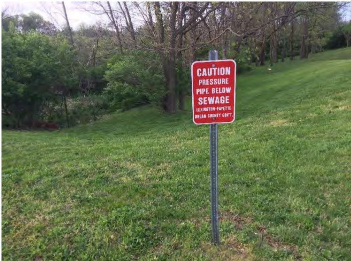
A2- Sewer Pressure Pipe Warning (b)
