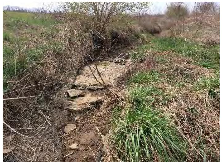
BI- Downstream End of Reach Facing Upstream
