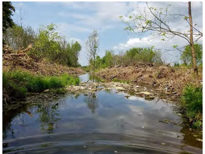
SITE 10 DOWNSTREAM VIEW OF CONSTRUCTION AREA
