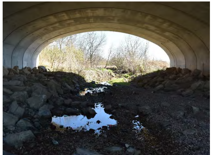
CR4- Looking Downstream Isolated Pools under Bridge
