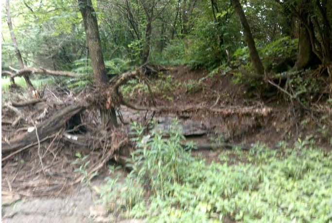
ES-4, Erosion and debris piles
