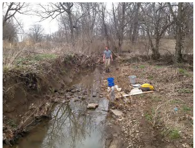
CR-8 Eroding Bank and Pool
