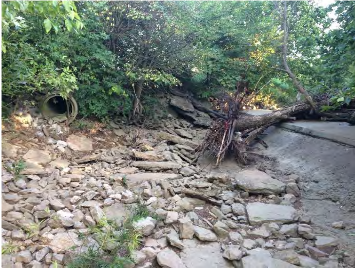
CRI - Effluent Pipe Stream Alteration
