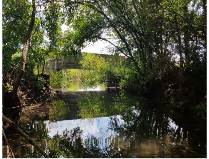
SITE 7 UPSTREAM VIEW OF ROAD CROSSING
