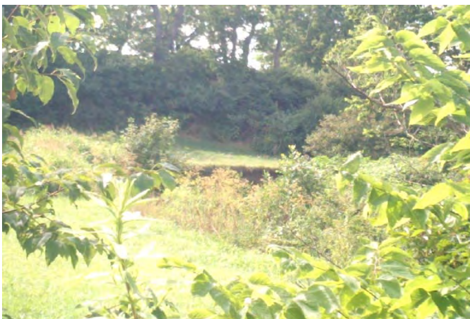
ES-8, Widening due to road crossing
