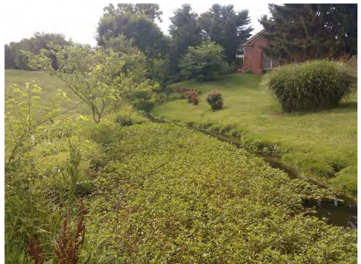
D4- Downstream View From Upstream End
