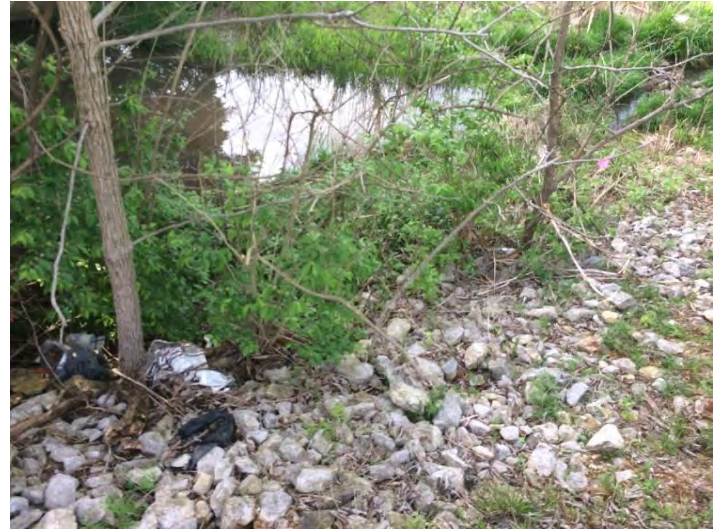
A2- Erosion Control on Rb of Reach
