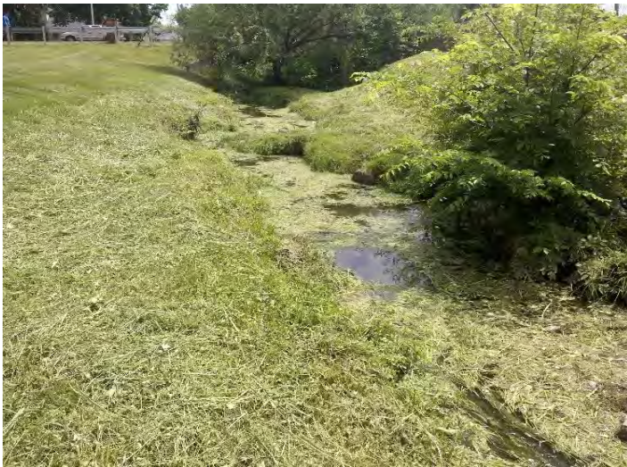
CR7- Upstream View from Upstream End
