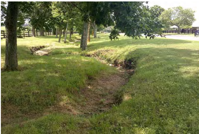
ES-7, Small erosion along narrow channel
