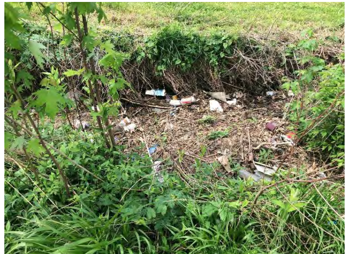
CR9- Undercut Bank Root Mat
