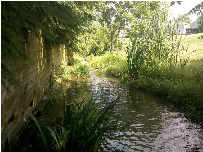
D4- Upstream View from Downstream End
