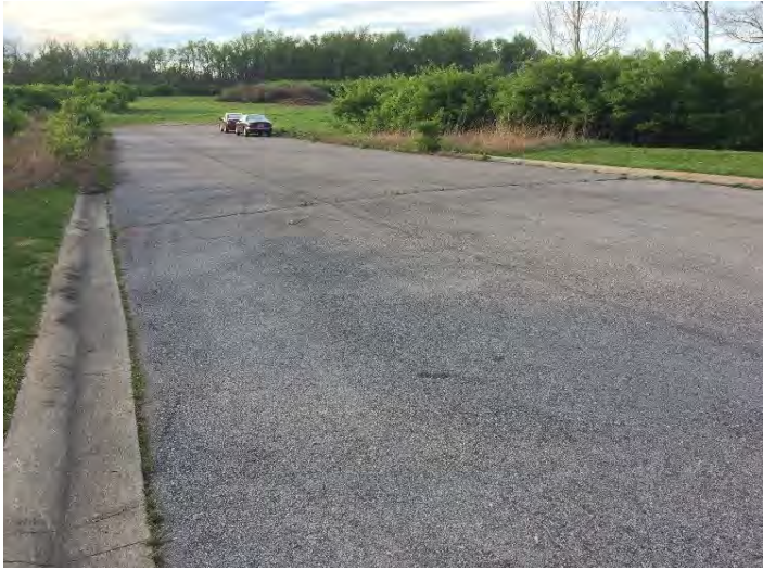
A2- Road above Culvert (b)
