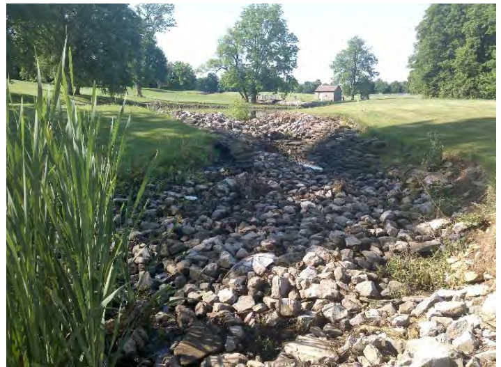
D3- Upstream view
