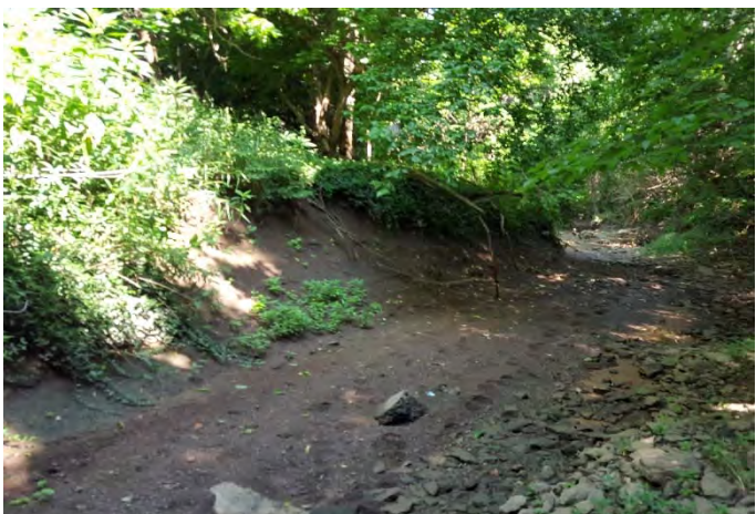
ES-6, Erosion of banks and heavy siltation
