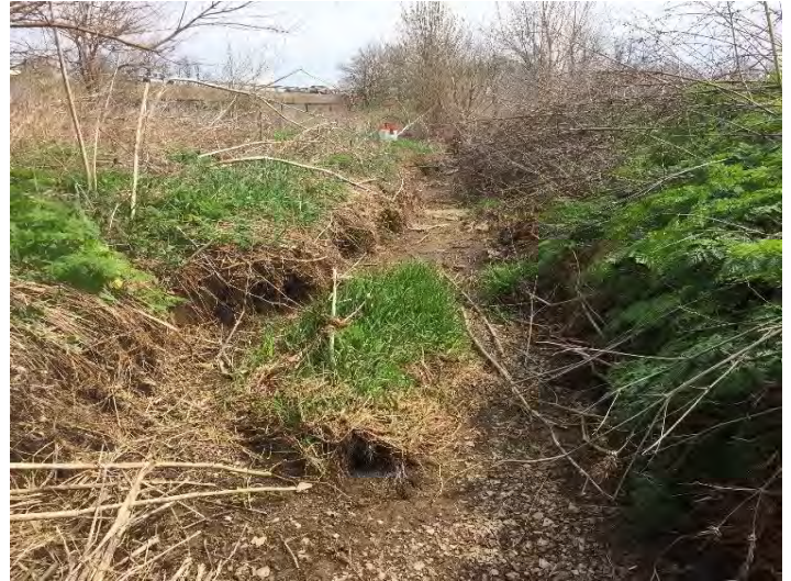
BI- Center of Reach Facing Downstream
