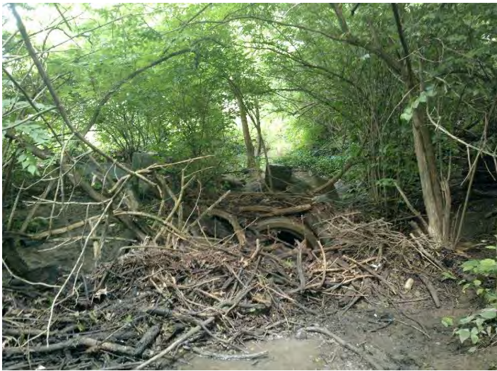
D5- Upstream View from Downstream End
