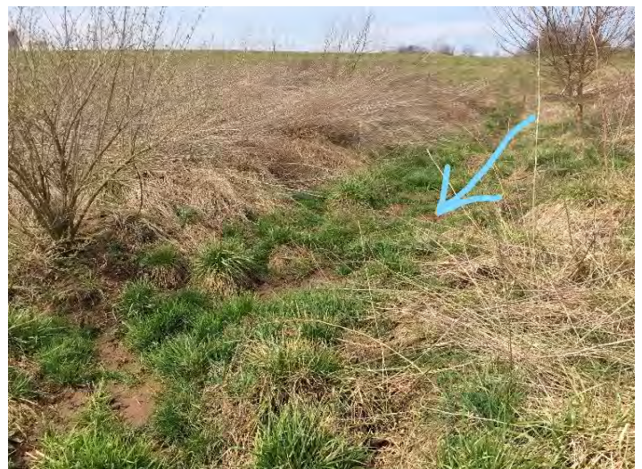
BI- Evidence of Drainage from Agriculture Field
