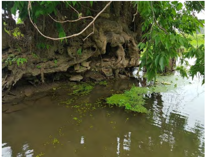
SITE 2 UNDERCUT BANK AND ROOT WADS
