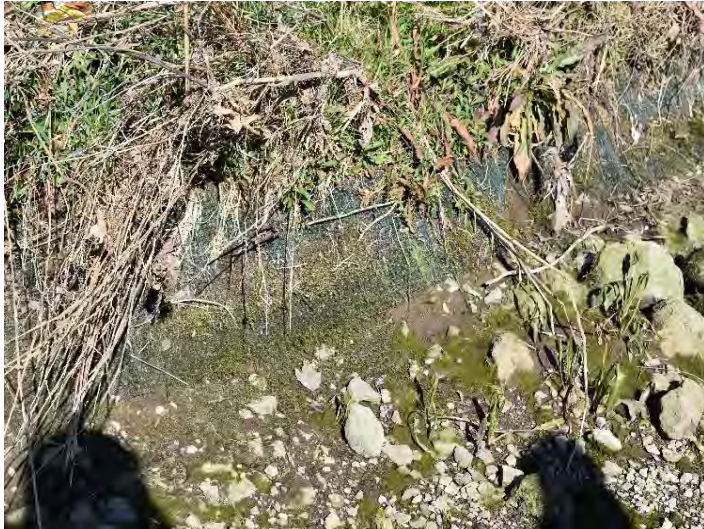
CR4- Bank Stabilization (a)
