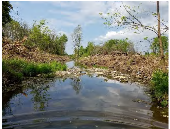
CR-5 Downstream View of Construction Area
