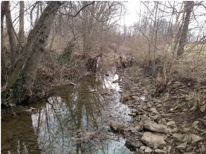
CR6- Upstream View from Downstream End of Reach
