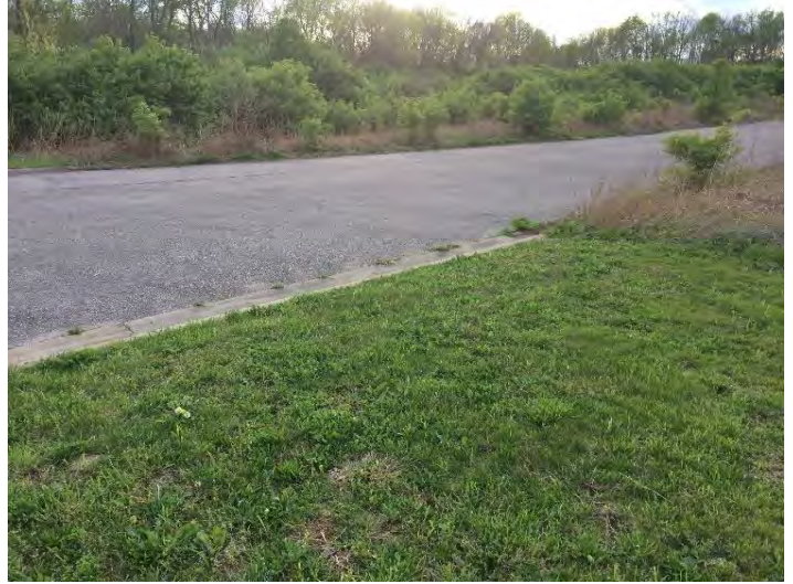
A2- Road above Culvert (a)
