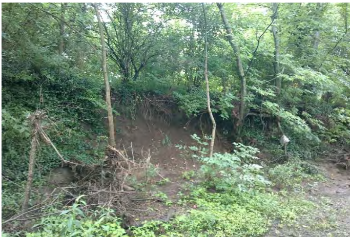
ES-2, Eroded bank about 6 ft tall
