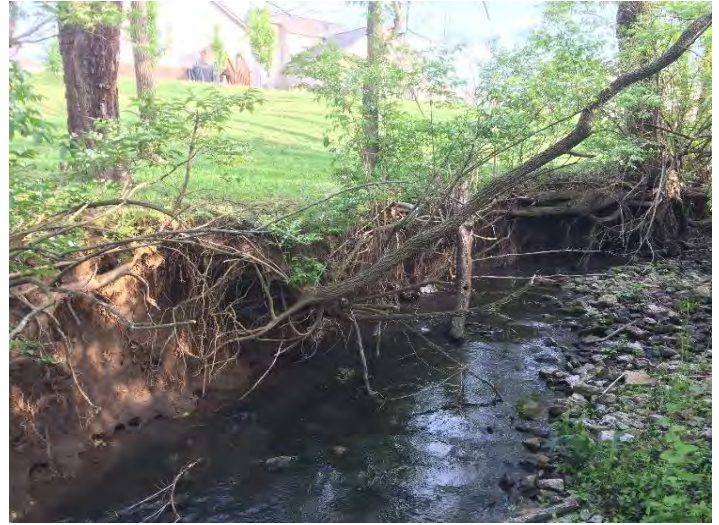
A2- Bank Undercuts (Rb) (a)
