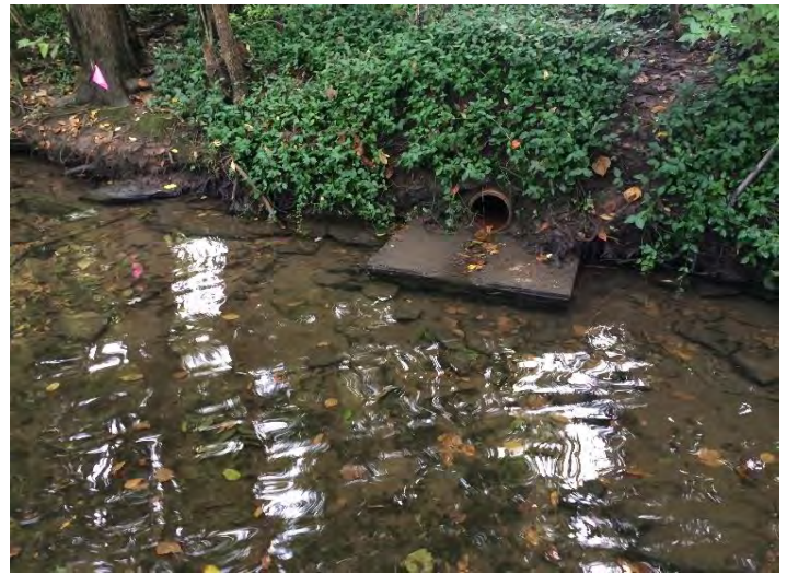
CR3 Effluent Pipe Upstream of Reach
