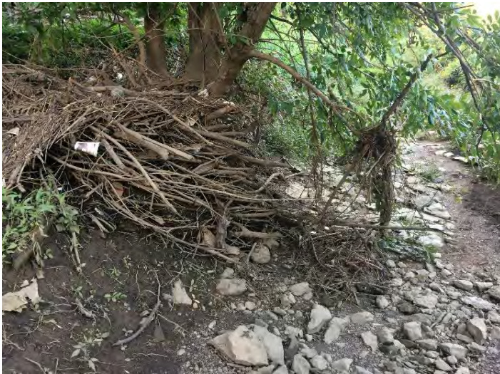
CRI- Undercut Bank Root Mat
