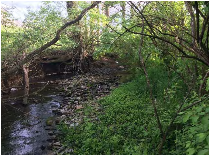
A2- Bank Undercuts (Rb) (b)
