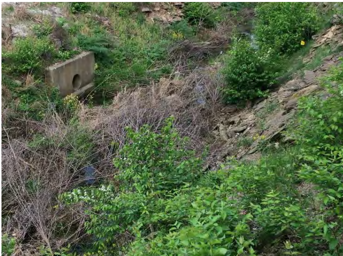
AI- Center of Reach, Culvert under I-64
