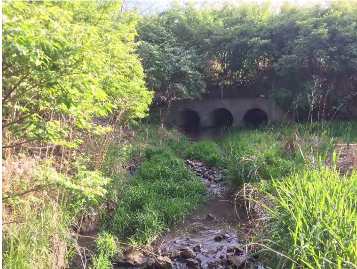
A2- Culvert Filter Facing Upstream
