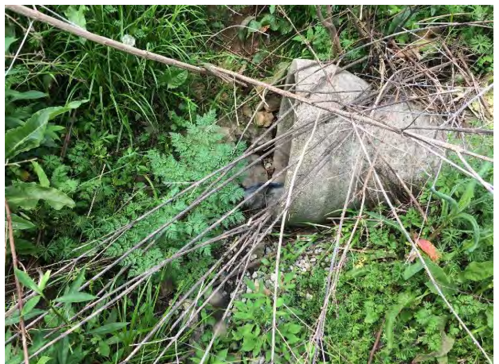
CR9- Culvert Downstream of Reach
