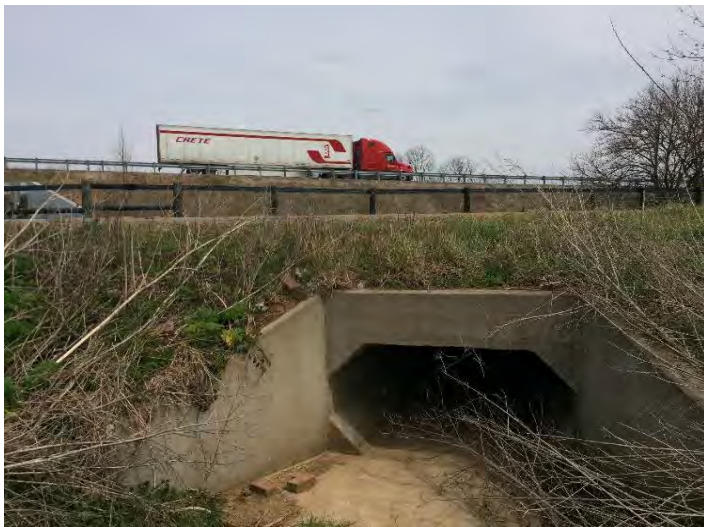
BI- Downstream End of Reach Facing Downstream
