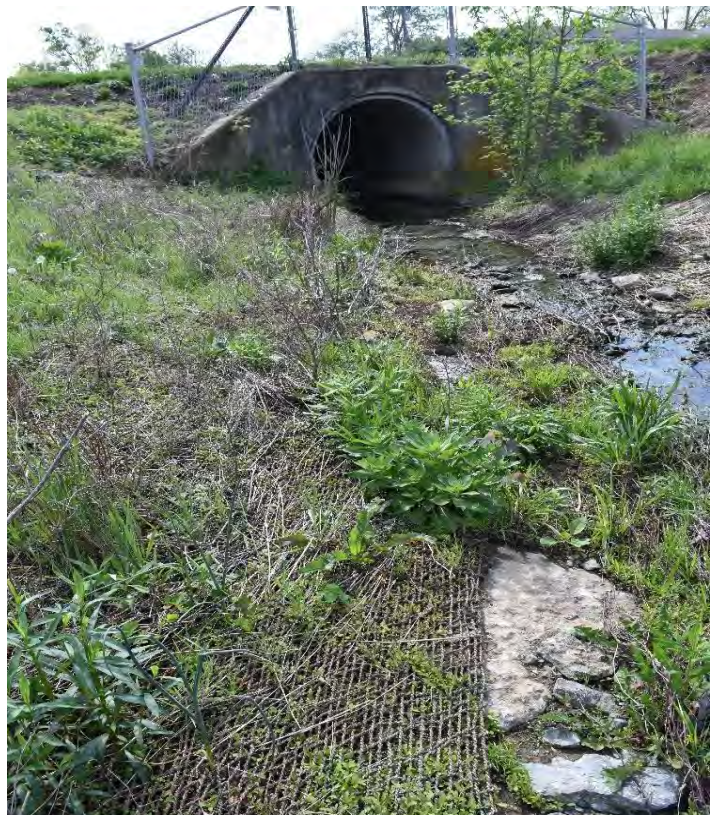
HI - Erosion Control Blankets
