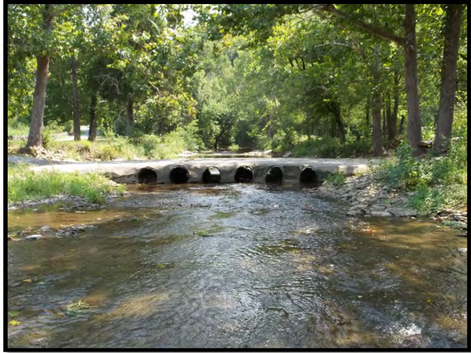
Figure 29. Site 3 Facing Downstream
