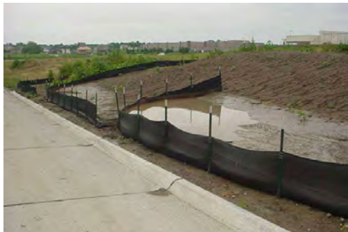
Silt Fence at Active Construction Site
