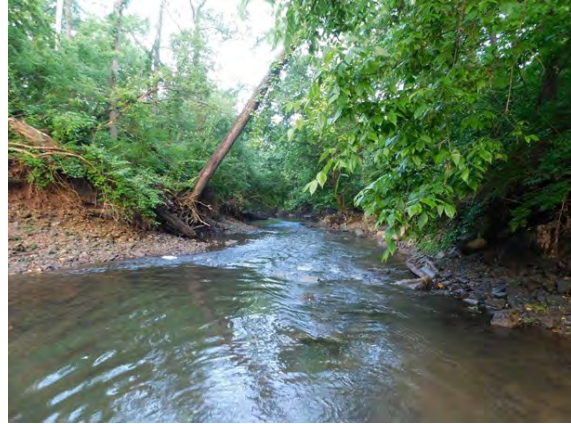
Figure 4.4 Looking downstream: stream bank and tree loss
