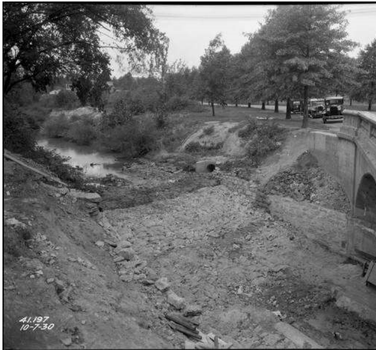
Figure 1.4 Sewer Construction at Beargrass Creek
