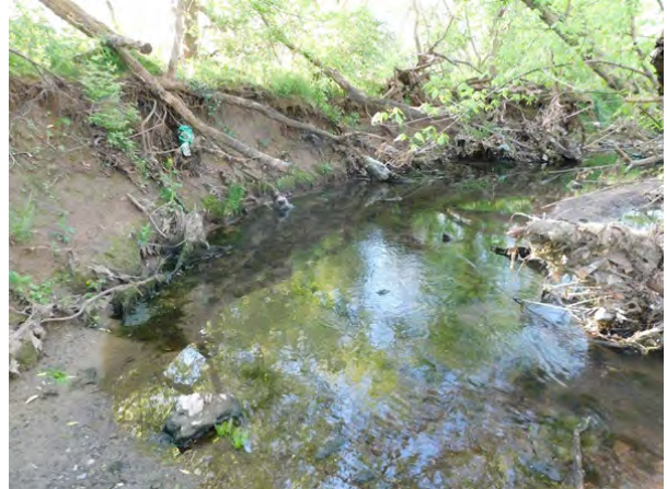
Figure 4.16 Looking downstream: bank vegetation loss and instability
