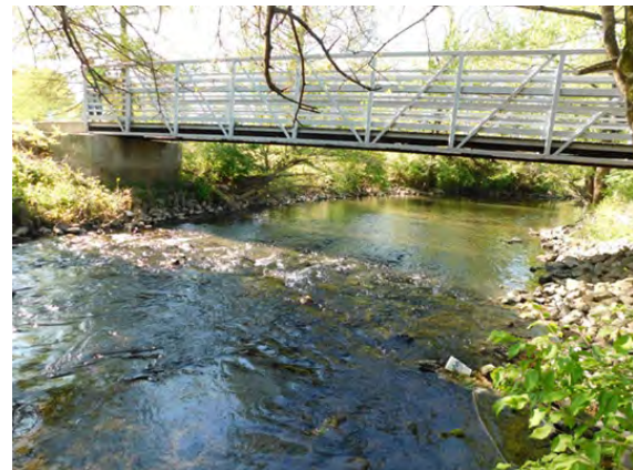
Figure 4.10 Looking downstream: pedestrian access north of Brown Park
